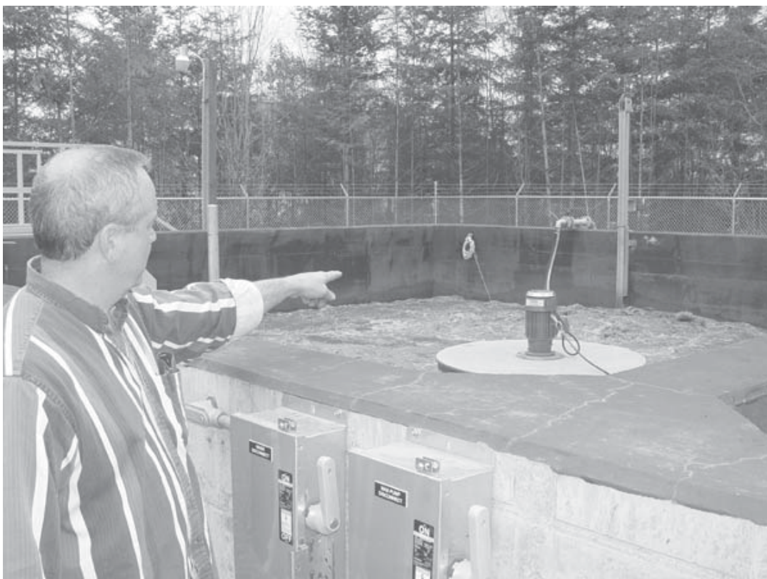
Utilities Specialist Bill Sherrill explains how the new treatment plant operates
